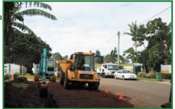
The town section of the pipeline is being laid along Lawyer Street and across Bunya Street down the back of the primary school then across paddocks to the pumping station. New pumps are also being installed at the pump station to handle to the extra demand.
